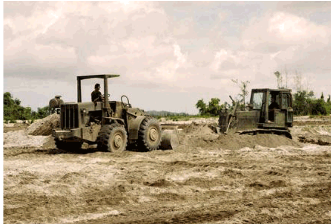
Seabees at Subic Bay and Cubi Point used a combination of a front loader and bulldozer to create berms of ash slurry before pushing it off to collection points for disposal. Photo taken October 19, 1991, Naval Station Subic Bay.
