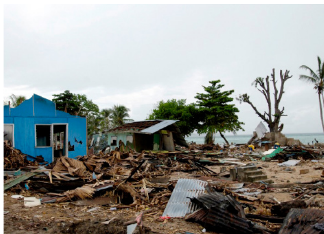
Houses destroyed by an earthquake and resulting tsunami on the Solomon Islands in April 2007.
