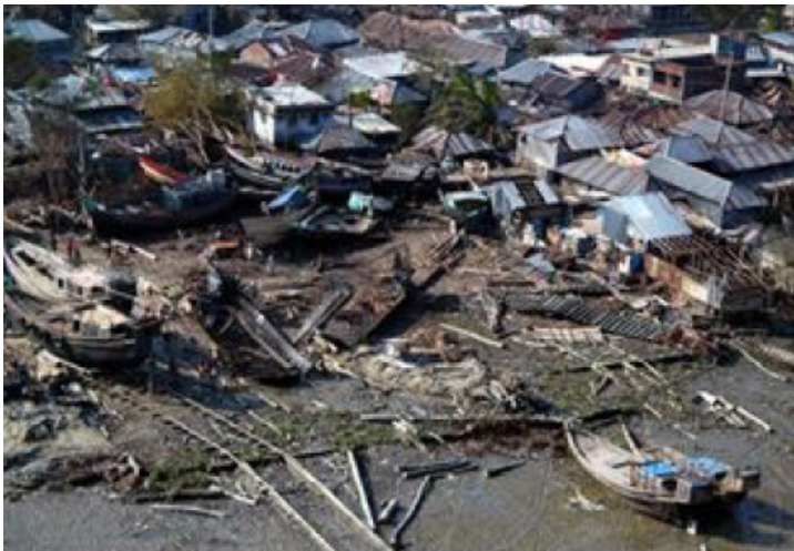
Aerial view of the destruction left behind by Tropical Cyclone Sidr in Bangladesh, Nov. 27, 2007. The USS Kearsarge and the embarked 22nd Marine Expeditionary Unit conducted humanitarian assistance and disaster relief missions.
