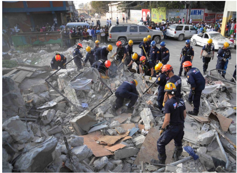
Members of the Los Angeles County Fire Department Search and Rescue Team clear debris at a collapsed building in downtown Port-au-Prince.
