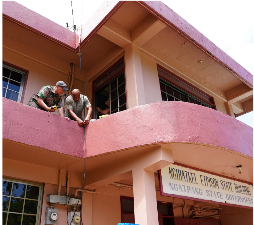
U.S. Marine Corps Lance Cpl. Ramon Jose Ceja, Combat Logistics Battalion 1, and U.S. Army Staff Sgt. Thomas Belanger, 1ST Theater Information Advantage Detachment, install an omni-directional antenna for an IC-M330 ICOM radio at the Ngiratkel Etipson State Building, Ngatpang, Palau, May 8, 2026. (U.S. Army photo by Staff Sgt. Mason Tran)
