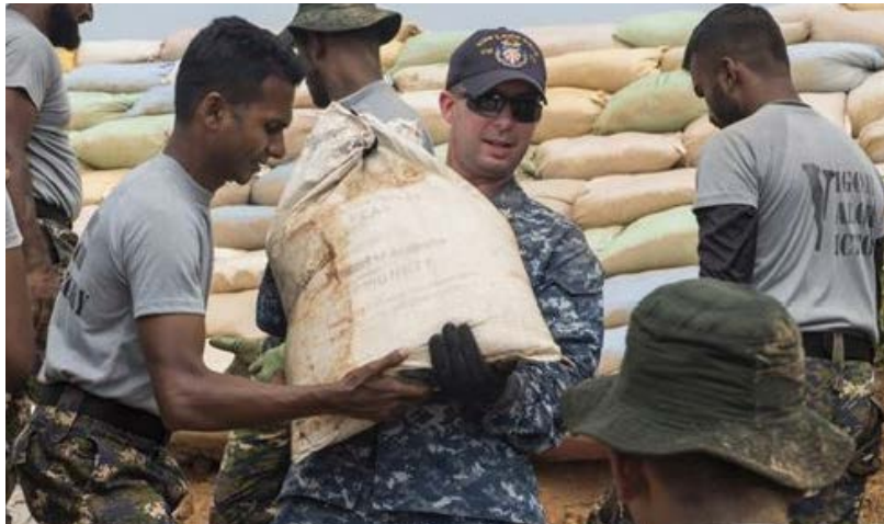
Fire Controlman 2nd Class Jason McEntire from the Ticonderoga-class guided-missile cruiser USS Lake Erie (CG 70) works with Sri Lankan Marines to repair levees in Matara, Sri Lanka, June 12, 2017 during humanitarian assistance operations in the wake of severe flooding and landslides that devastated many regions of the country. U.S. Navy photo by Mass Communication Specialist 2nd Class Joshua Fulton Source: https://www.pacom.mil/Media/News/News-Article-View/Article/1211414/uss-lake-erie-us-servicemembers-render-assistance-in-sri-lanka-after-devastati/
