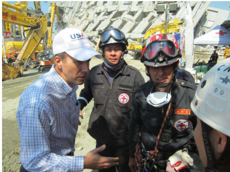
USAID/OFDA Regional Advisor Brian Heidel and Taiwan Red Cross staff survey earthquake damage in Taiwan's Tainan city. (American Institute in Taiwan)
