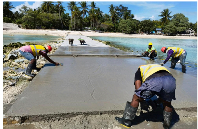
Figure 10. Bridge Construction in Kiribati (Xinhua, 2022)
